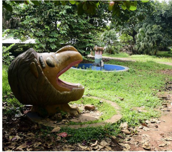
At work: The Lions Park being renovated under AMRUT-2 by Kozhikode Corporation in 2023. FILE PHOTO States and cities.
